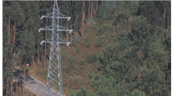
Helicopter view of a 60kV overhead line crossing a densely forested area.
